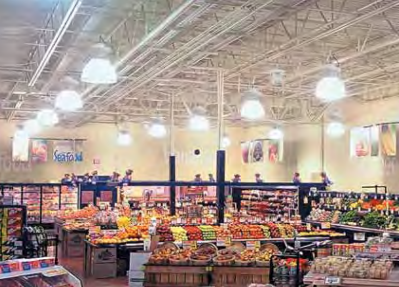
Figure 2. While HID electronic ballasts can save energy, they are especially useful for applications requiring good color stability, such as this grocery store. Photo courtesy of GE Lighting.
